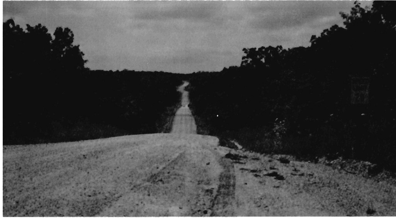
Route W, looking west from Route I, is an all weather gravel road typical of loose-surface roads on the reservation. Note irregular, undefined shoulders and concrete ford (Ford 41) in background.
