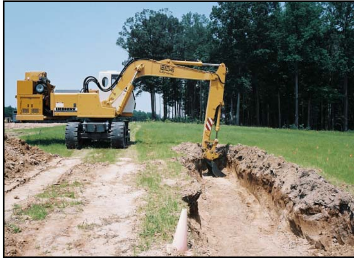
Figure 7. Working Across Trench
