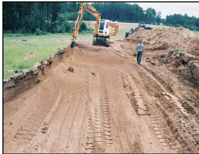
Figure 12. Vertical Mill Completing a Rearward Pass
