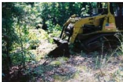
Picture 46 – Bucket moving debris
