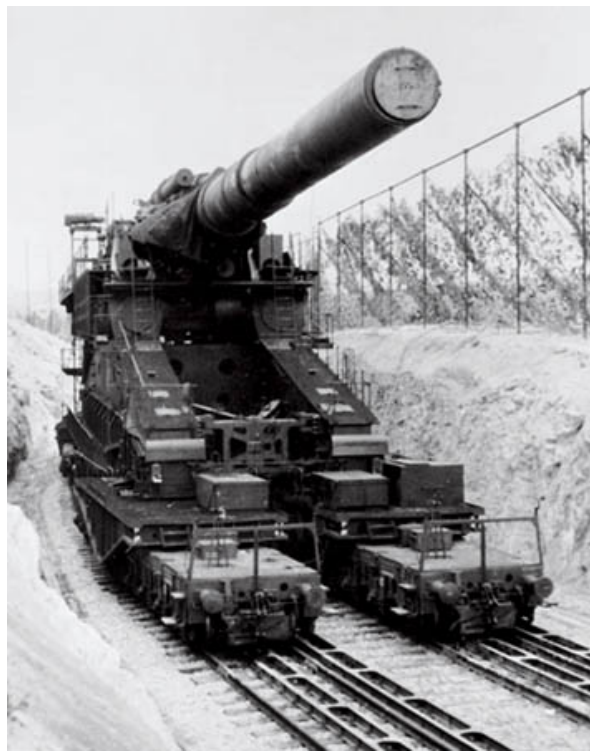
Figure 1. The German Gustav Gun was so large special railroad tracks had to be laid to move the weapon (From Eisenstein, 2004).
