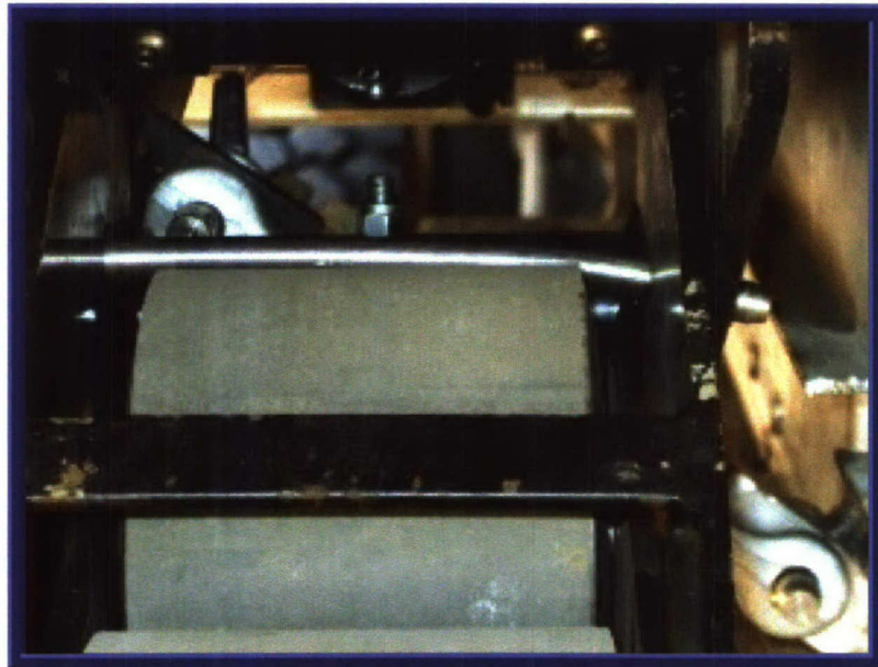
Photo 1. Bent Roller Pin
