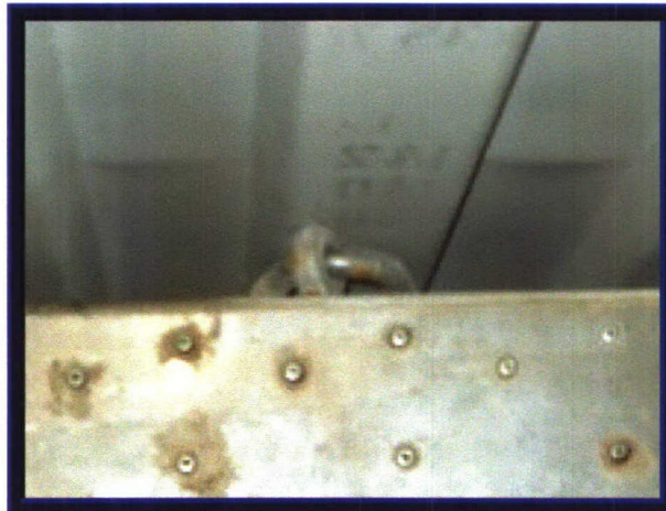
Photo 13. Contact of Tiedown with Container Wall.
