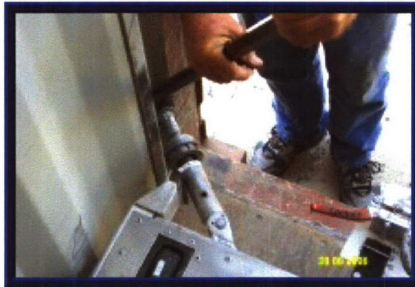
Photo 12. Disengagement of Corner Lock of JMIP with Tools.
