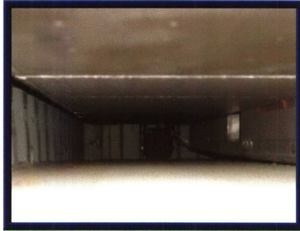
Photo 6. Rollers Holding the Main Rails off of the Container Floor.
