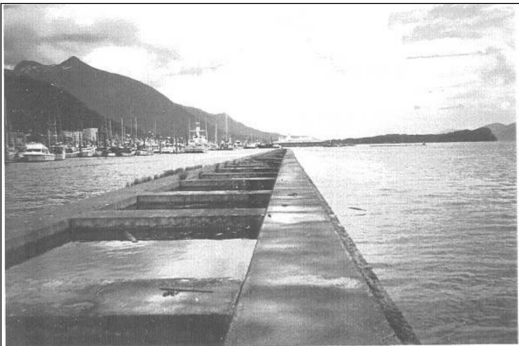
Bar Point Harbor Large Breakwater (#1)
