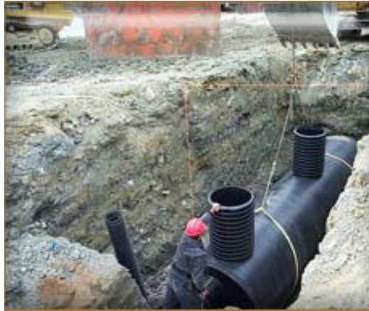
Figure 5: Installing an Oil-Water Separator (SD1, 2006).
