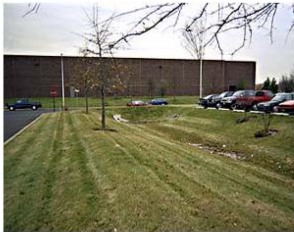
Figure 11: Grassed Swale Photo (EPA, 2006a). Grassed swales can be used along roadsides, parking lots, and buildings to collect and treat stormwater runoff.
