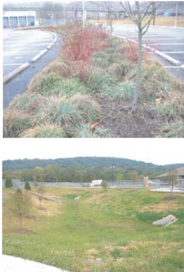
Figure 7: Biofiltration Swale and Dry Detention Basin Retrofit (SD1, 2006). Sanitation District No. 1 in Fort Wright, Kentucky retrofitted their existing administrative office facility with numerous structural BMPs to serve as an example for the community.
