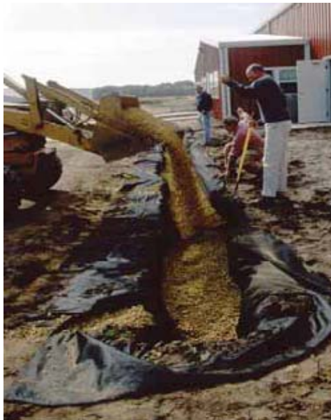
Figure 9: Infiltration Trench Construction (PWUD, 2006). Infiltration trenches are first lined with filter fabric and are then back-filled with stone to capture pollutants as the water filters down to the soil.
