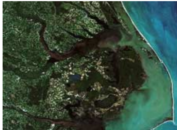
Figure 5.3 North Carolina coast after Hurricane Floyd
