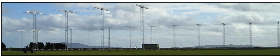
Fig. 8 TIGER Unwin Antennas. 16 element transmit/receive antenna (background) and 4 element receive only antenna (foreground) [Courtesy M. .
