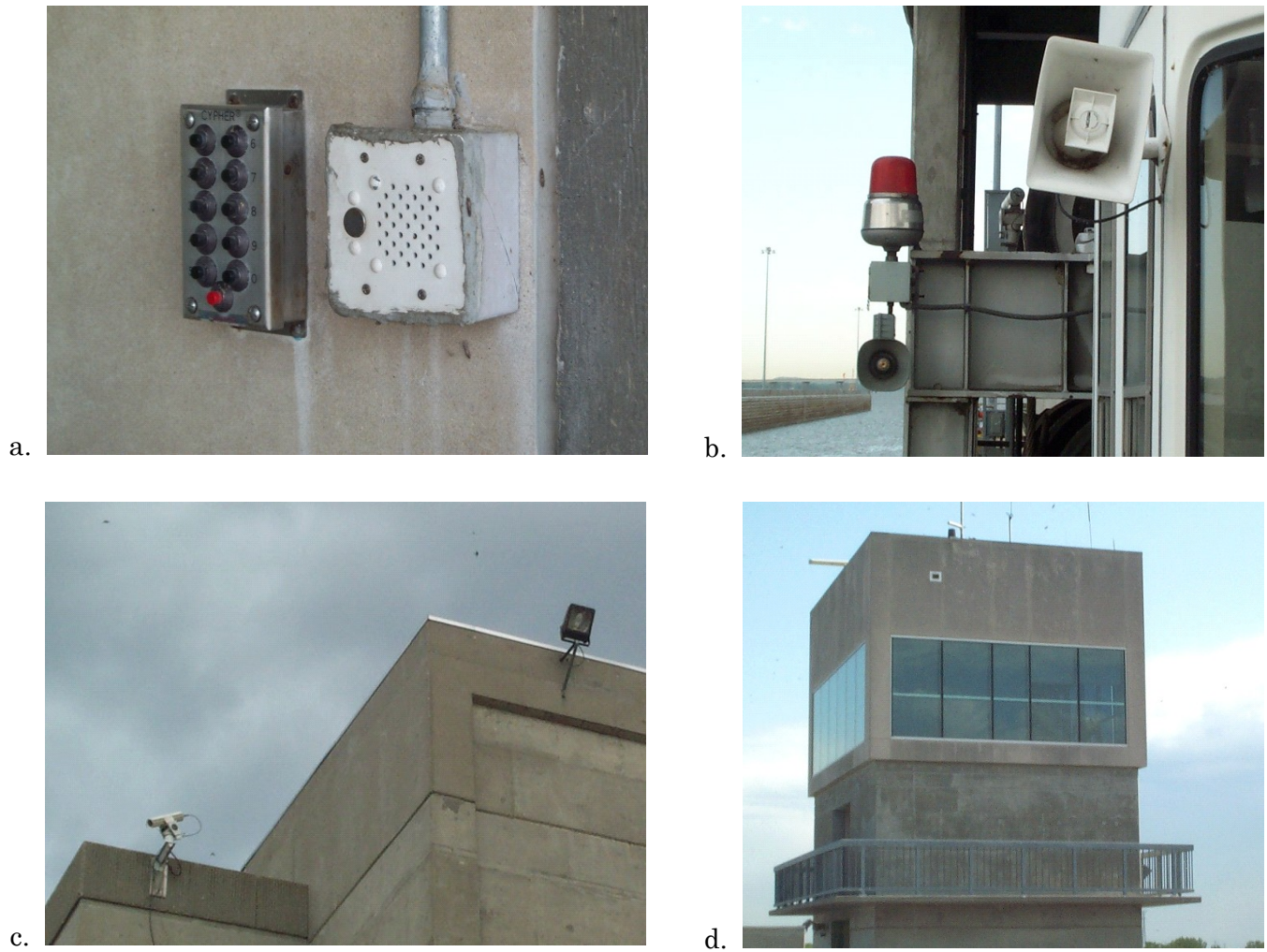
Figure 6.3. Lock and dam security measures, including coded locks (a), intercom and alarm systems (b), closed-circuit cameras and lighting systems (c) and observation tower (d).
