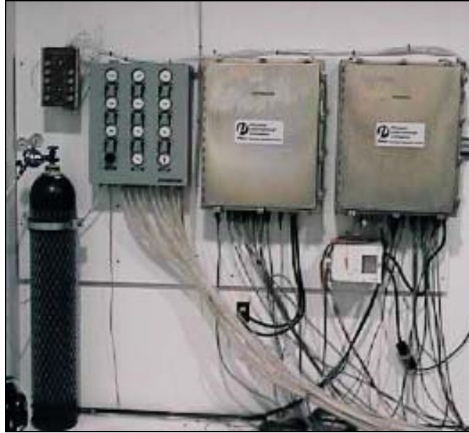
Figure 9. Dry gas bottle and its distribution panel, interlock box, and interface J-box (left to right).
