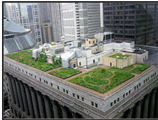
Figure 2.3. 22,000 Square-Foot Rooftop Garden on Chicago City Hall (US DOE, 2007).
