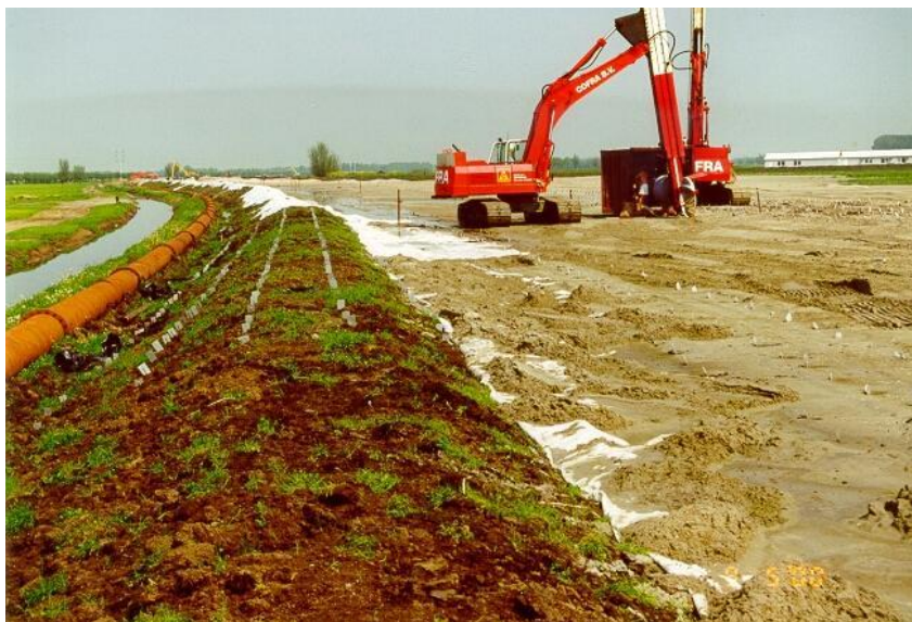
Figure 76 Inserting vertical strip drains to decrease pore pressure
