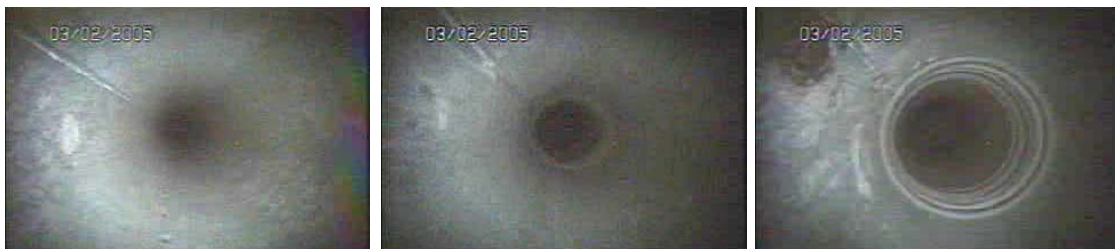
Figure 10. Pipe interior following grit blast.
