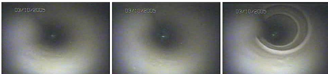
Figure 11. Interior of pipe following epoxy lining.
