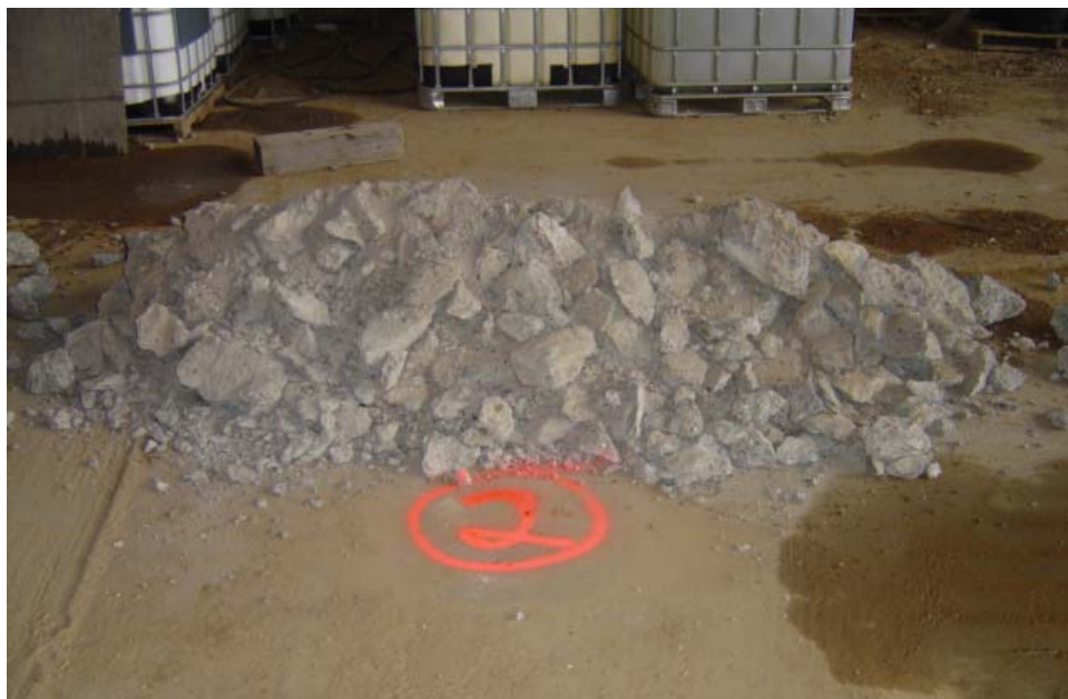
Photo 19. The RCP material removed from Repair 2
