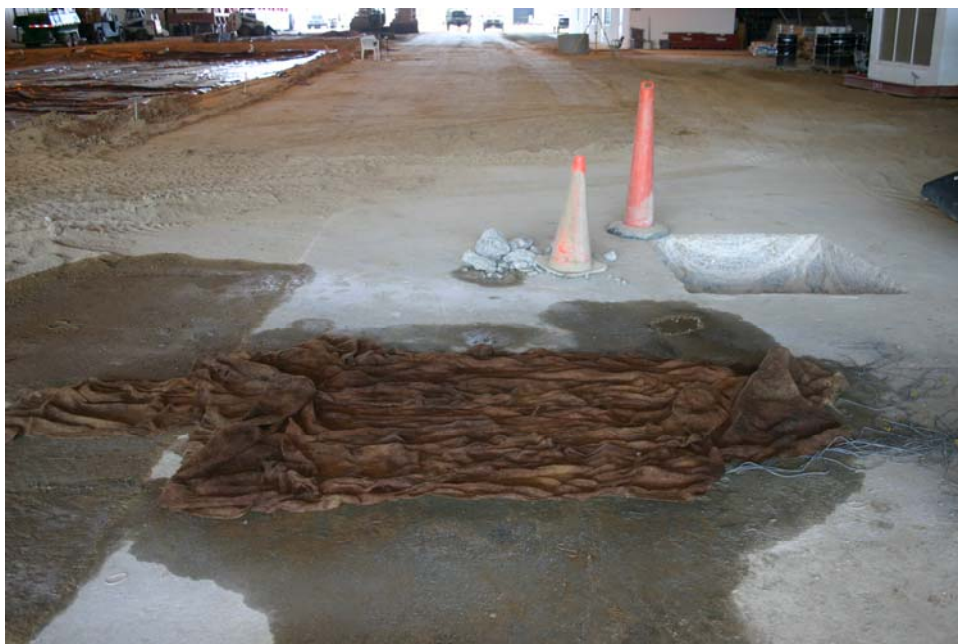
Photo 26. Moist curing of Type III grout using soaked burlap
