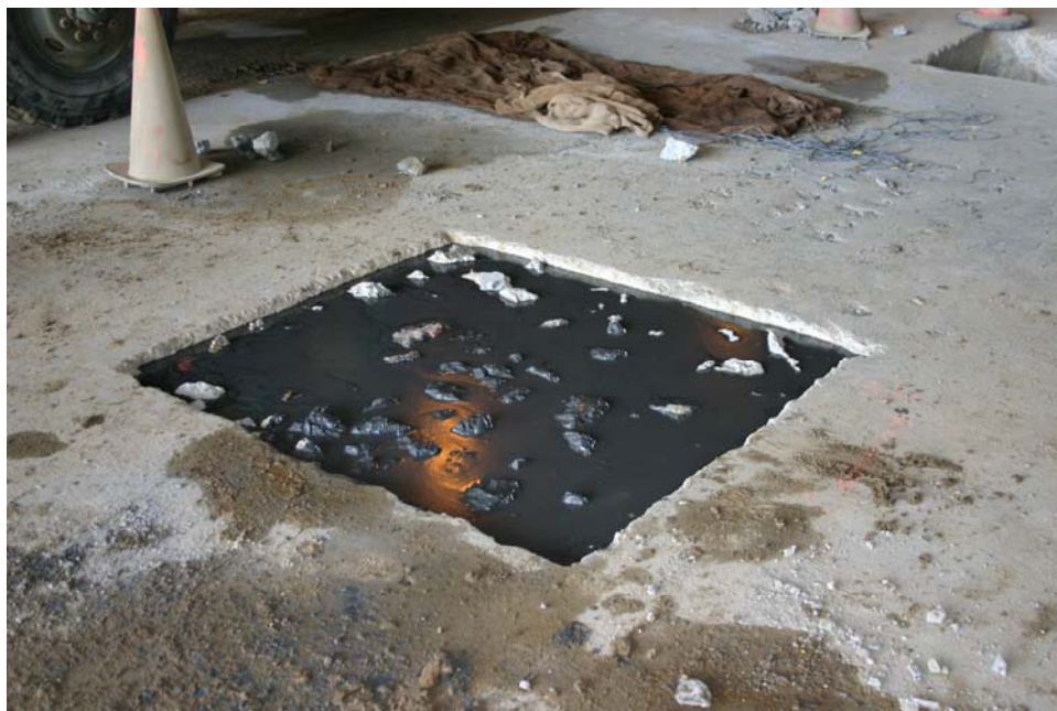
Photo 29. Pavemend™ repair just prior to pouring the final lift
