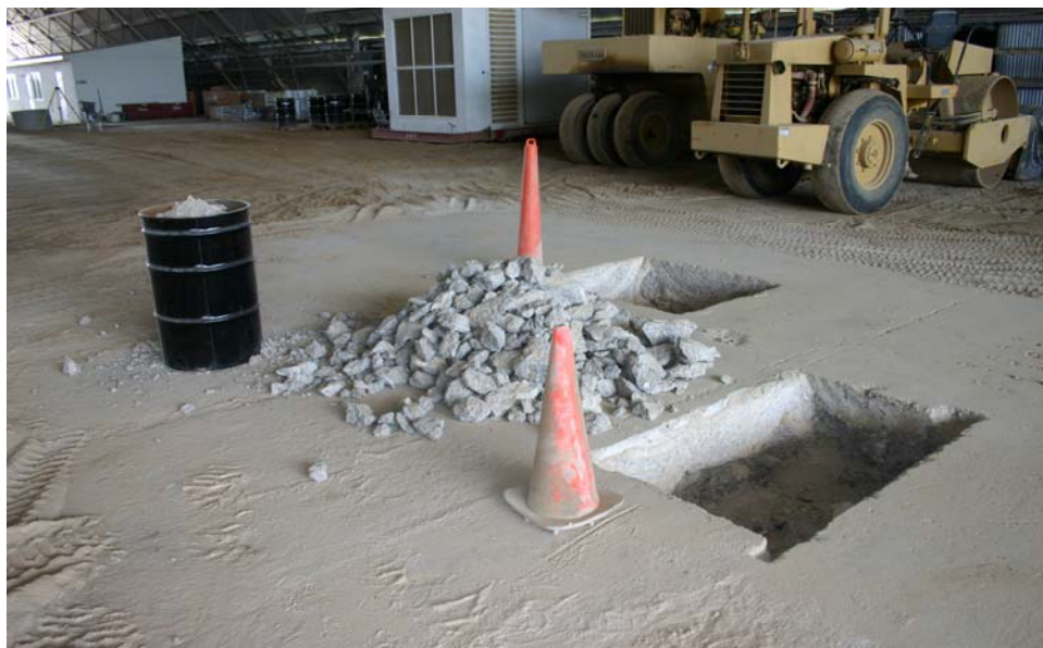
Photo 20. Unusable material screened into large container (black drum)
