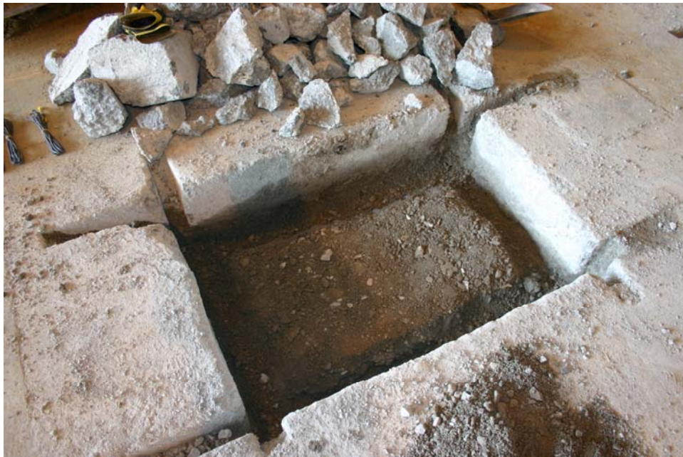
Photo 21. Repair 8 with thickened edge prior to RCP placement
