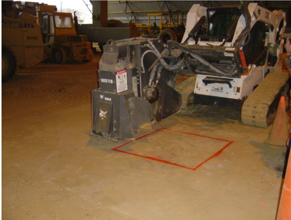
Photo 15. The outline of the repair marked with fluorescent paint
