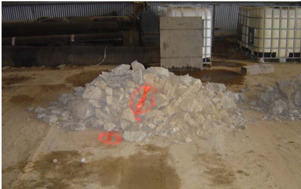
Photo 1. RCP material after demolition and excavation from the repair hole
