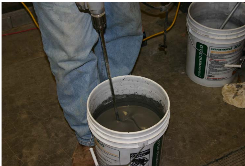
Photo 3. Mixing a single batch of Pavemend™ in its own container with a drill and paddle mixer
