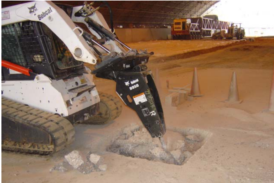
Photo 16. Pavement breaker attachment breaking the interior of the repair
