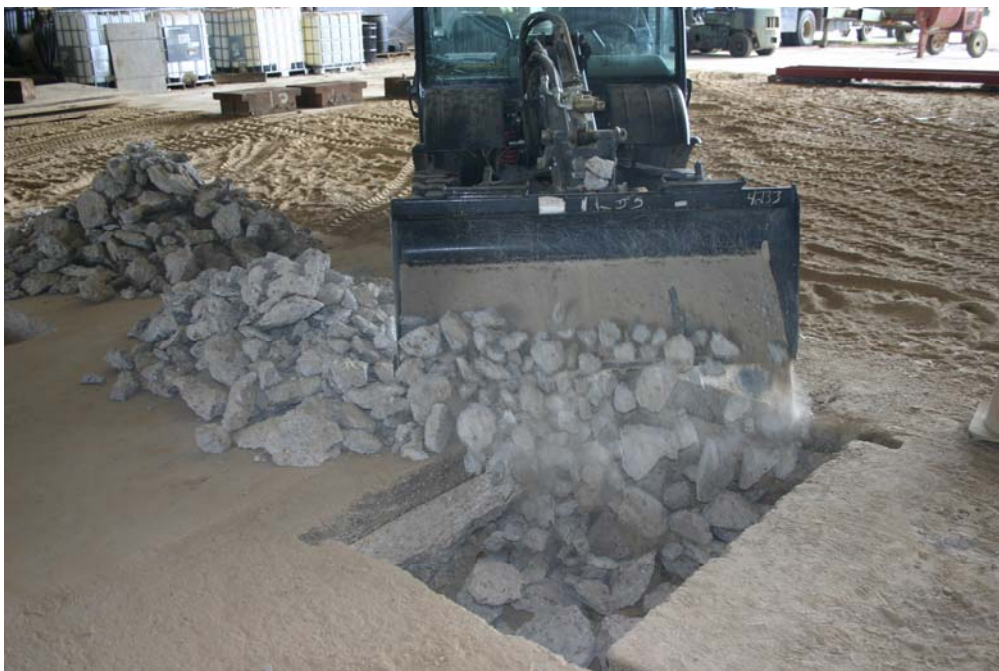
Photo 23. Placement of the RCP into the repair
