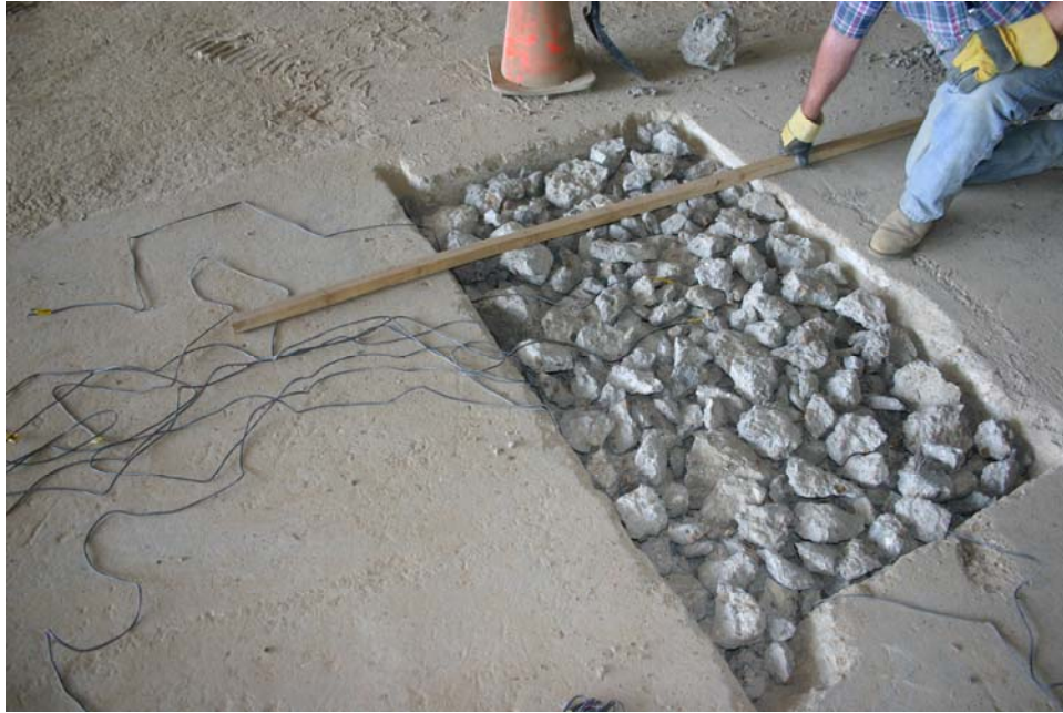
Photo 24. Checking the surface of the repair area to ensure there is no protruding material
