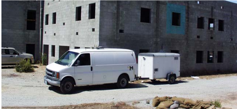
Figure 2 Photograph of Instrumentation Van
