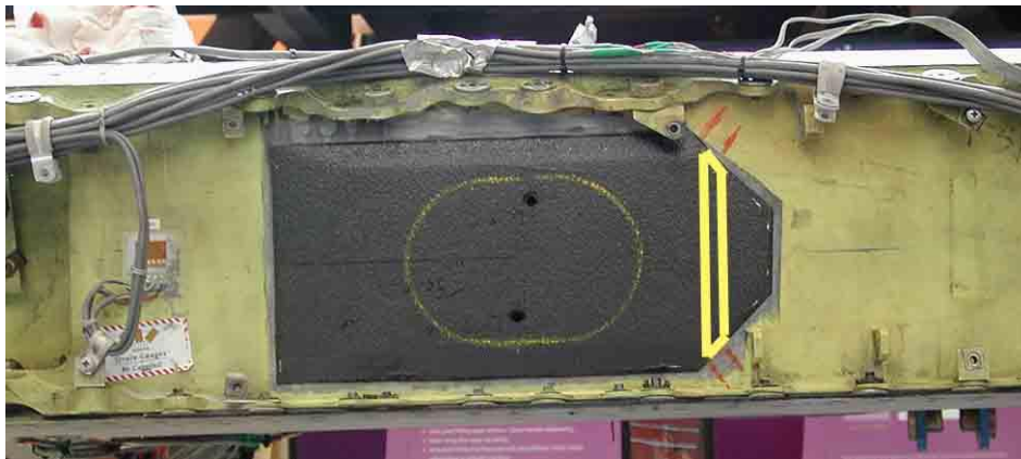
Figure 10: Boron Doubler Repair at Opening in Forward Spar at FSS 163
