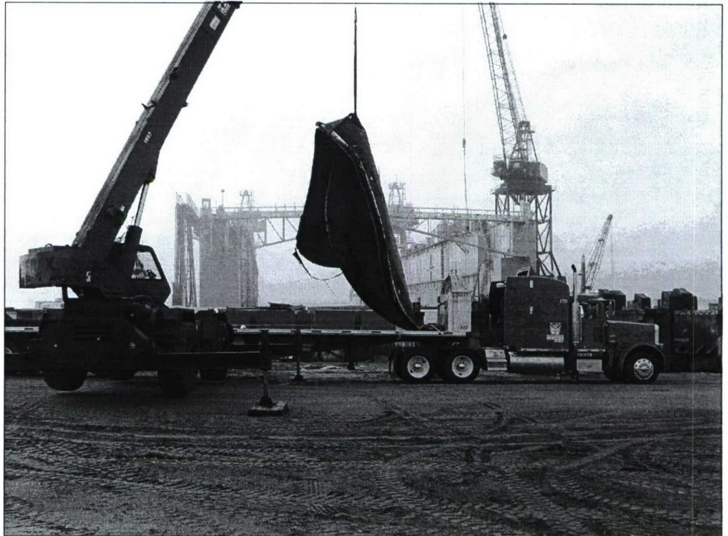
The sonar dome assembly is lowered onto the truck by the crane. The dome is a rubber and metal composite weighing 20,720 pounds that was cut in half and hauled away on two semi-trucks.
