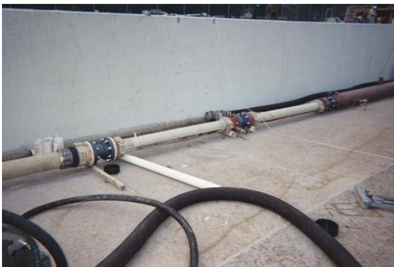
Figure 12. Installation of Tandem Streaming Current Sections
