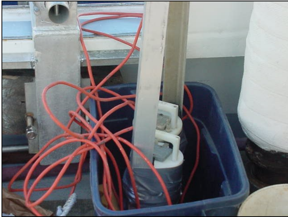
Figure 7. Water-level gage mounted on angle iron.
