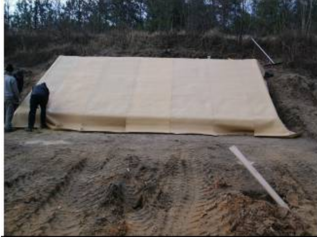
Figure 28. Seams of Top Rubber Cover Sealed.
