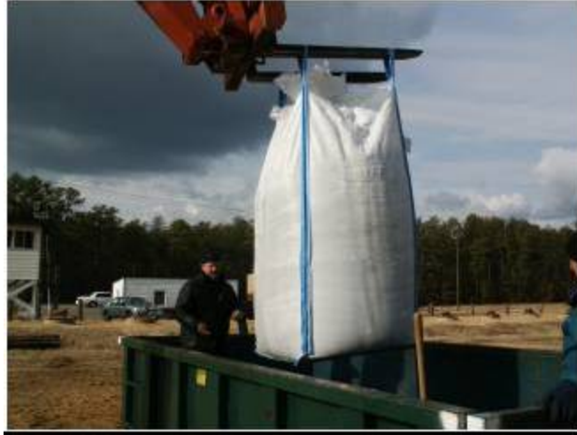
Figure 20. Emptying Super-Sacs of Granular Rubber.
