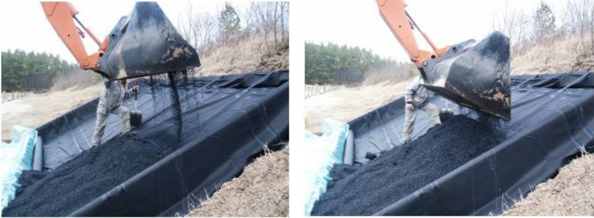
Figures 22 and 23. Adding Granular Rubber into the Bullet Catcher Frame.
