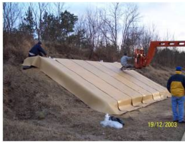
Figure 27. Sealing the Seams of the Top Rubber Cover.
