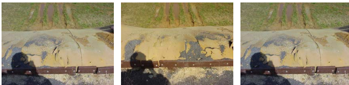
Figures 38, 39, and 40. Damage to the Upper Portion of the Top Rubber Cover of the Range 5 Bullet Catcher.
