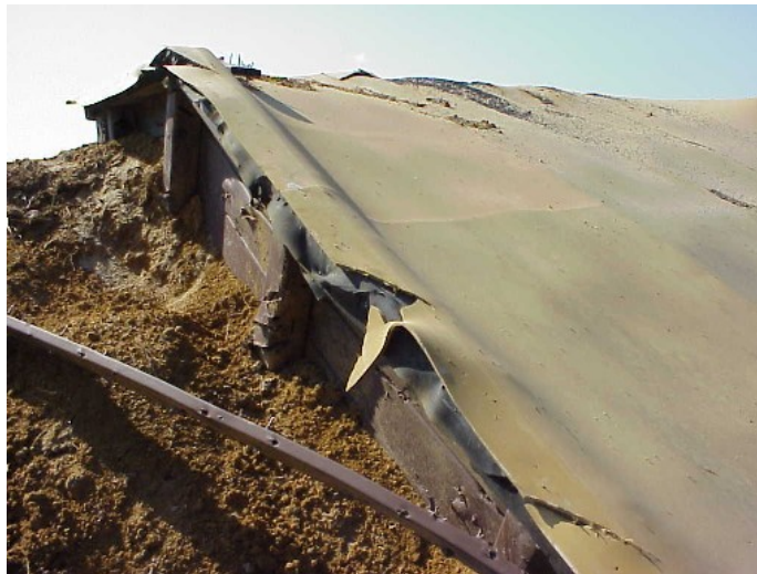
Figure 37. Left Side Damage to Top Rubber Cover and Frame/Planking on Range 5.
