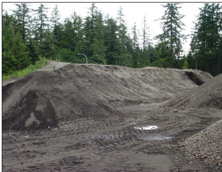
Figure 51. Partially excavated Evergreen Range Berm.
