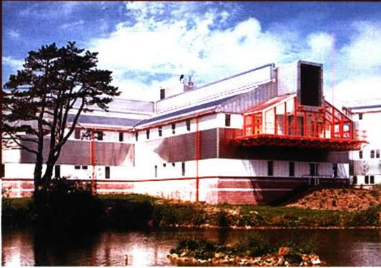
EXTERIOR VIEW FROM LAKE SHOWS USE OF MATERIALS AND STEEL CLADDING FOR SOLAR GAIN. PHOTO FROM WWW.ABK.CO.UK .
