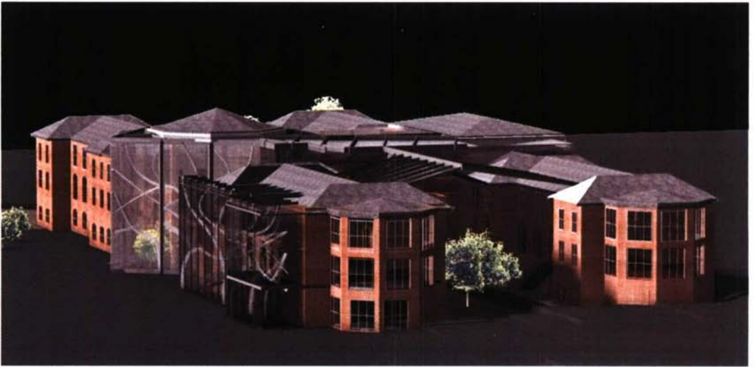
NEW GLASS CIRCULATION STRUCTURE WRAPS NEW EAST FACING FACADE
