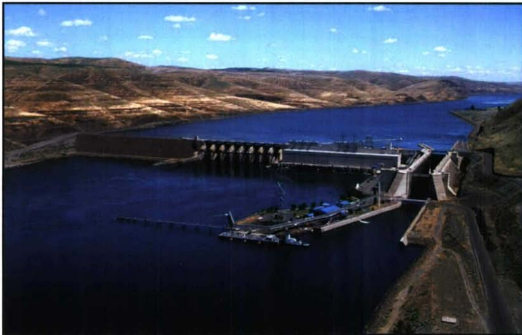
Little Goose Lock and Dam Starbuck, Washington
