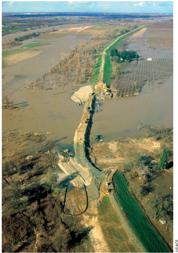
A breached levee along the Sacramento River, California, is being repaired.
