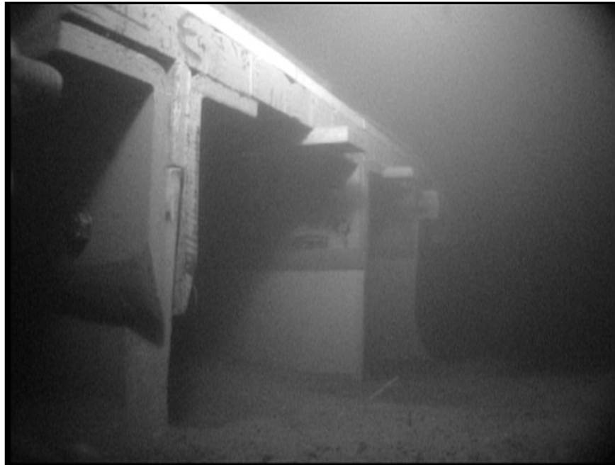
Figure 8. Image of the aft embedment plates, showing that the depth of embedment was not uniform for all plates.
