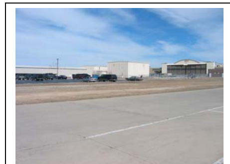
Figure 2-1. The new Squadron Operations Facility would be located in this area south of Building 700 under the Proposed Action (photo taken facing northeast).
