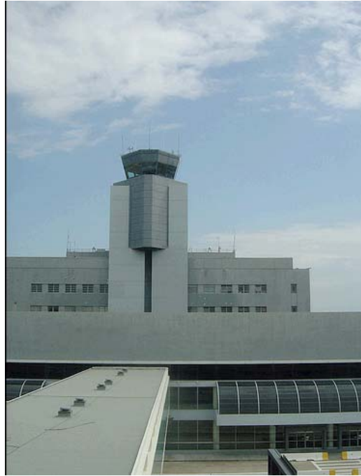
SFO Control Tower
