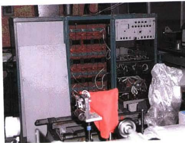
Fig. 24. The general view of the power supplier
