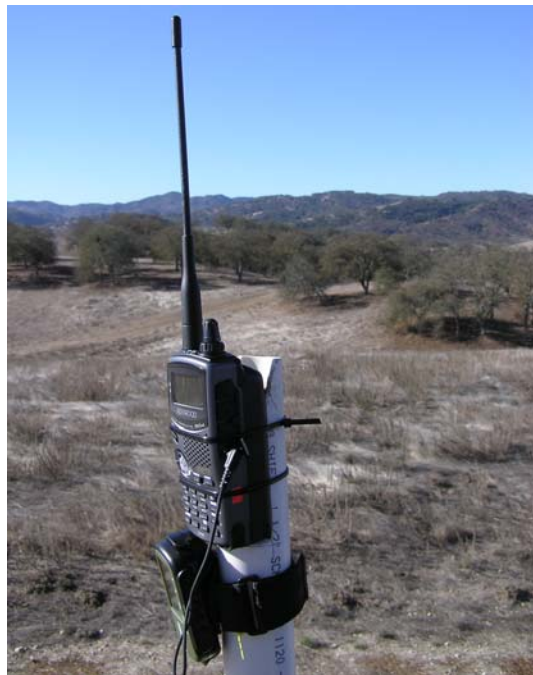
Figure 31. APRS transceiver on a pole.
