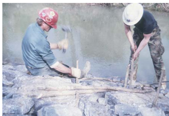
Figure 3. Installing a joint planting
