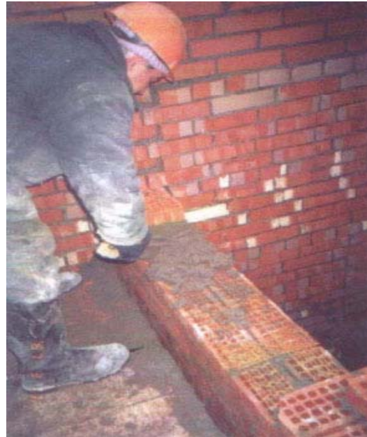
Fig. 5. Using of perforated steel band as reinforcement:
