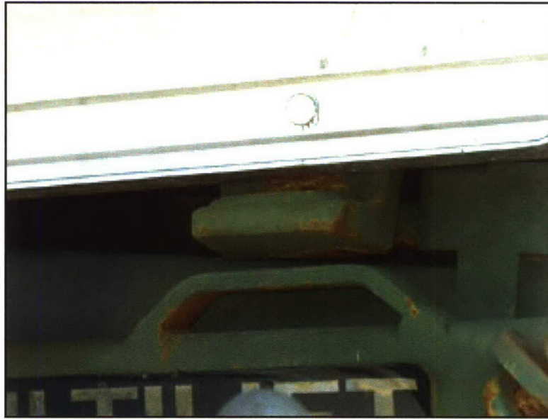
Photo 10. JMIP Rails not on PLS Truck Supports
