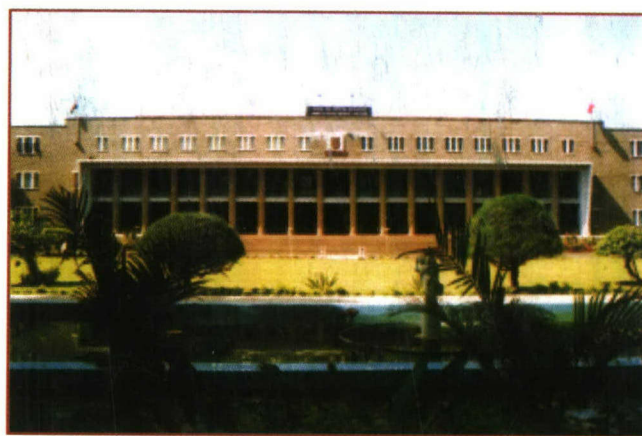
AFMC – One of Pune’s most notable architectural landmarks
