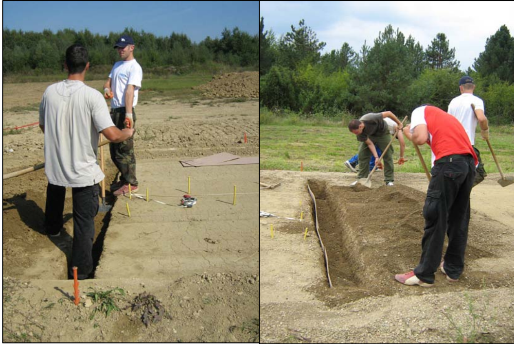
Figure A-10. Witness Board Installation
