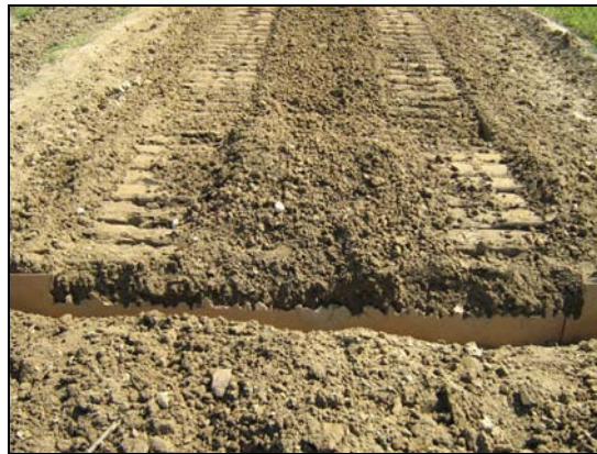
Figure A-11. Witness Board Partially Excavated
