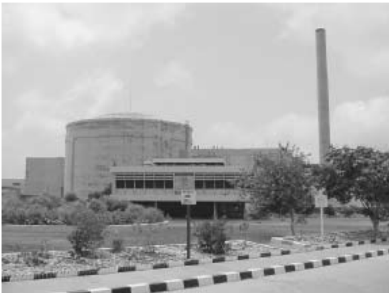
Figure 1. The Karachi Nuclear Power Plant (KANUPP).
