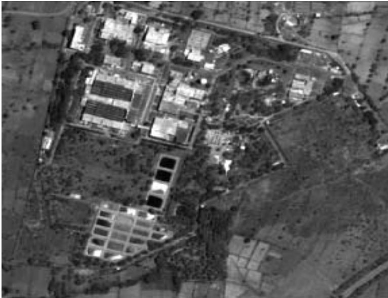
Figure 5. The Centrifuge Enrichment Plant at Rattehalli, Mysore. 54
