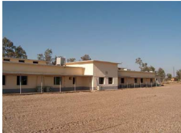
Office Building in Battalion Area After Reconstruction
