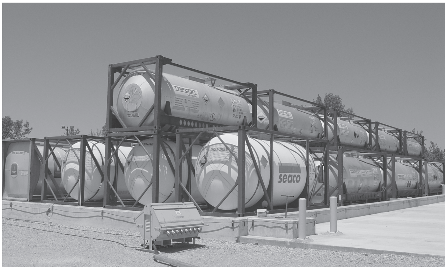
Figure 4: Intermodal Storage Containers at the Newport Chemical Agent Disposal Facility, Newport Chemical Depot, Indiana
