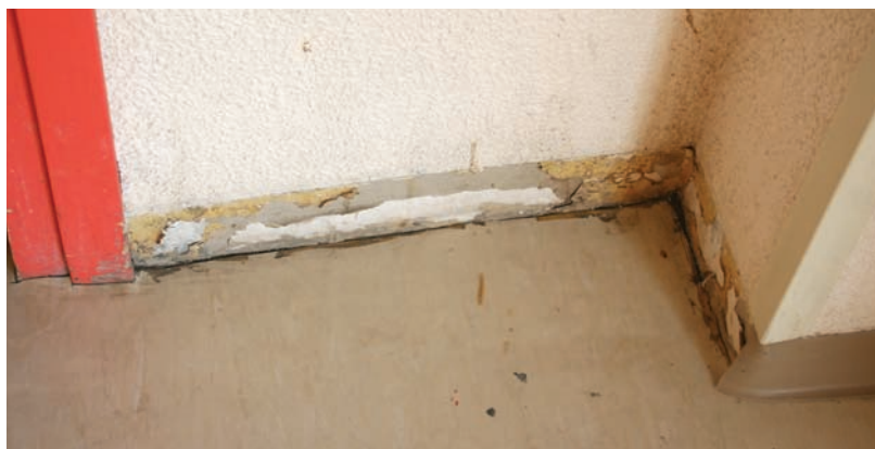
Water saturated and damaged wall with visible mold.
