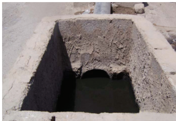
Newly constructed manhole. (Photo courtesy of USACE)
