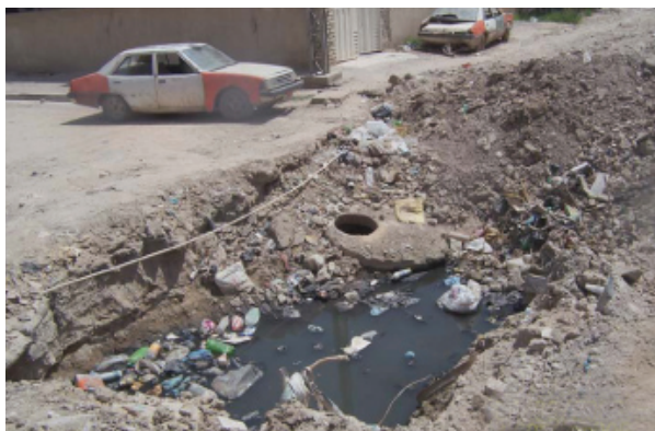
Collapsed existing manhole before construction completed by the contractor. (Photo courtesy of USACE)
