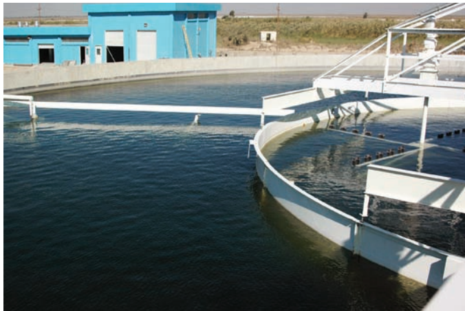
Refurbished water treatment plant.
