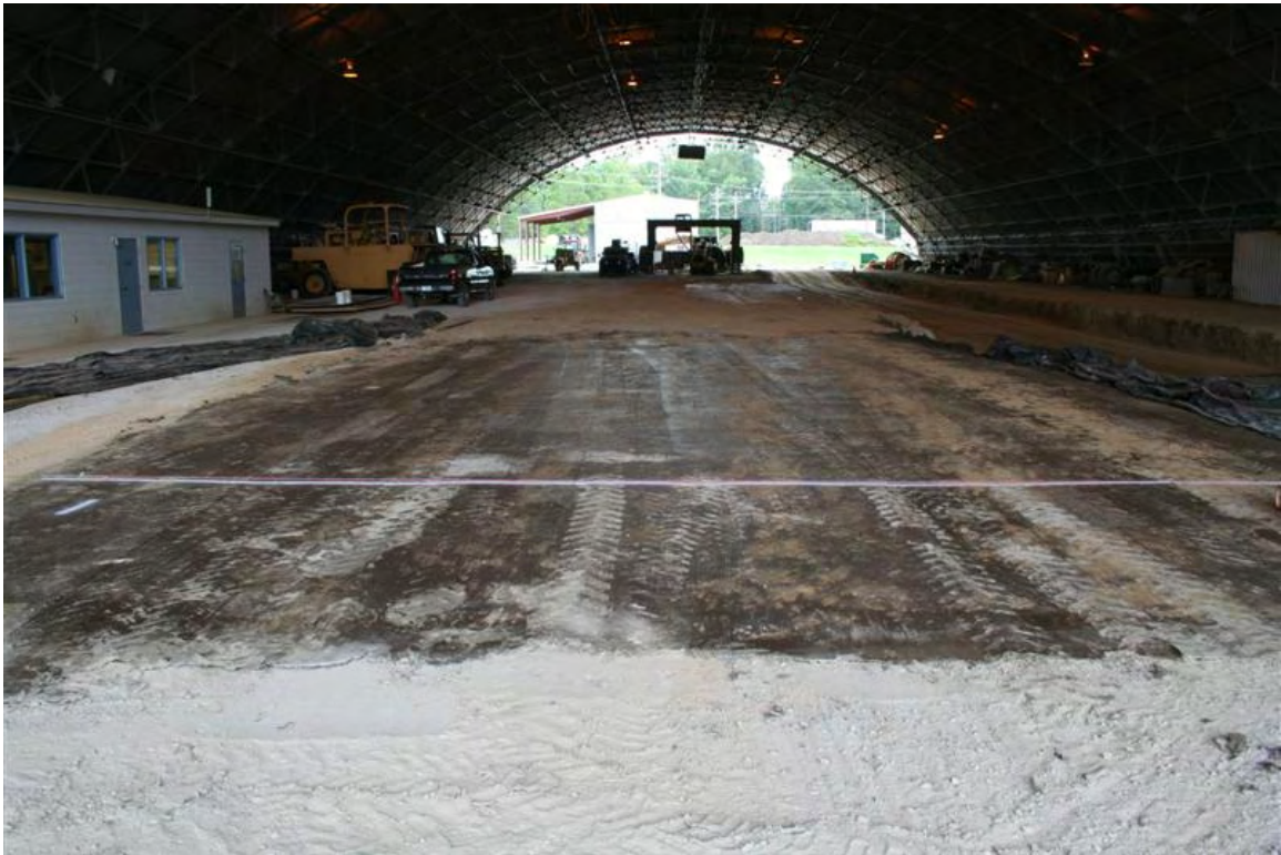
Photo 17. CH Material Test Section Prior to Installation of DURA-BASE® Mat
