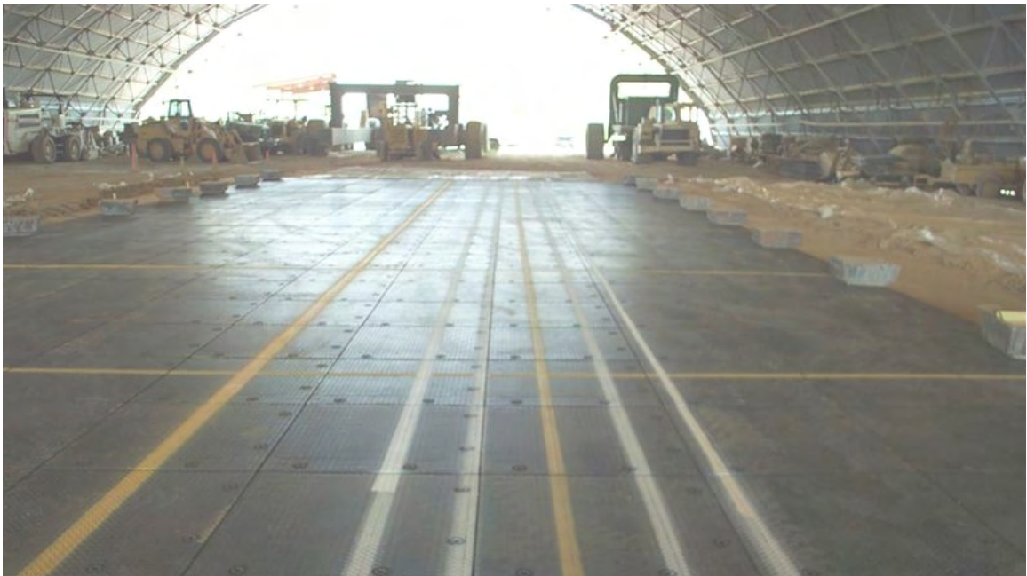
Photo 19. Bravo® Matting Striped and Ready for Traffic – Lead Weights on Sides Used as Edge Anchors
