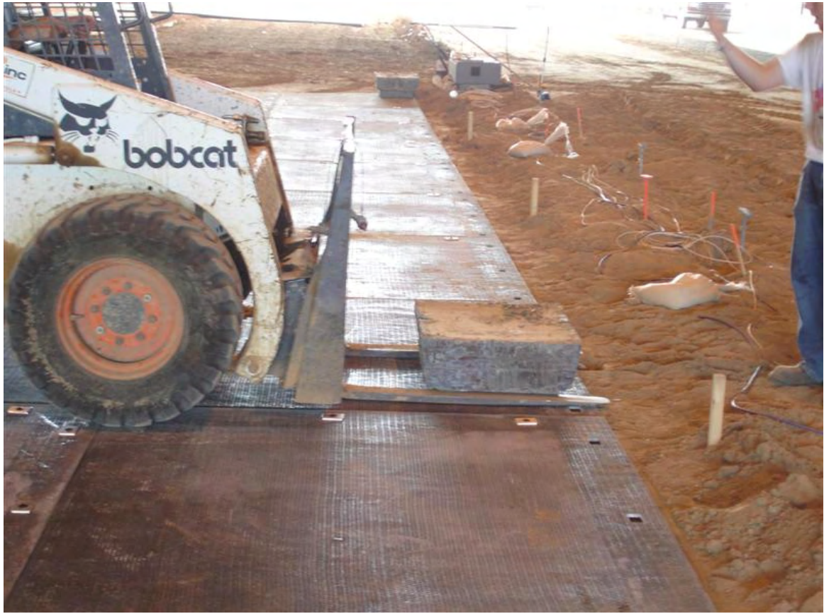
Photo 20. Placement of 907-kg (2,000-lb) Lead Weight on Edge of ACE-Mat™
