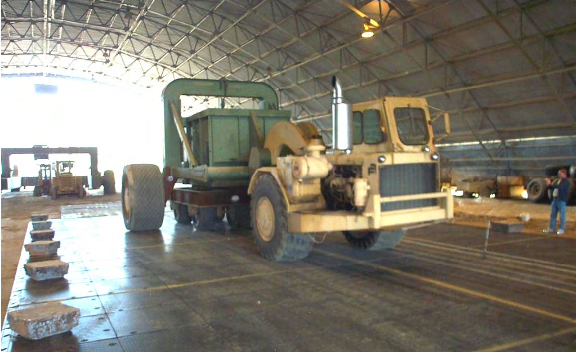
Photo 32. Trafficking on the BRAVO® Mat on SM Test Section
