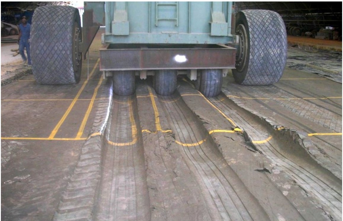
Photo 28. High Plasticity Clay (CH) Control Test Section After Rutting Failure (1 Pass)
