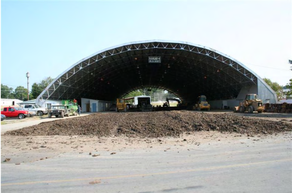
Photo 5. Hangar 4 Test Facility at ERDC in Vicksburg, Mississippi in 2007
