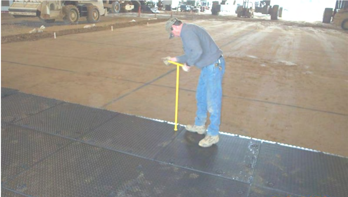
Photo 10. Turning the Pin in a Bravo® Mat to Lock It in Place
