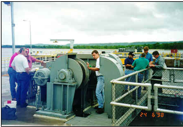
Illustration 12. Lock and dam operating equipment.
