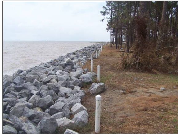
Figure 13. Bank line revetment structure.
