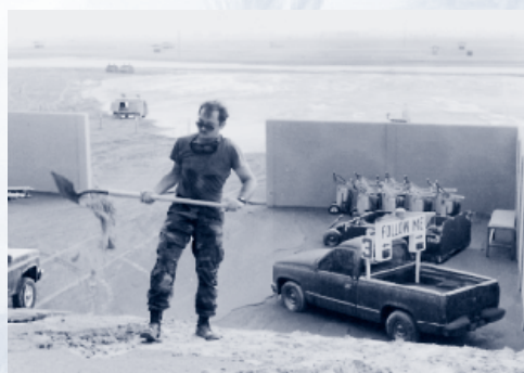
The first priority of clean up was to shovel the roofs clear of tons of ash to make safe the work and living areas.
