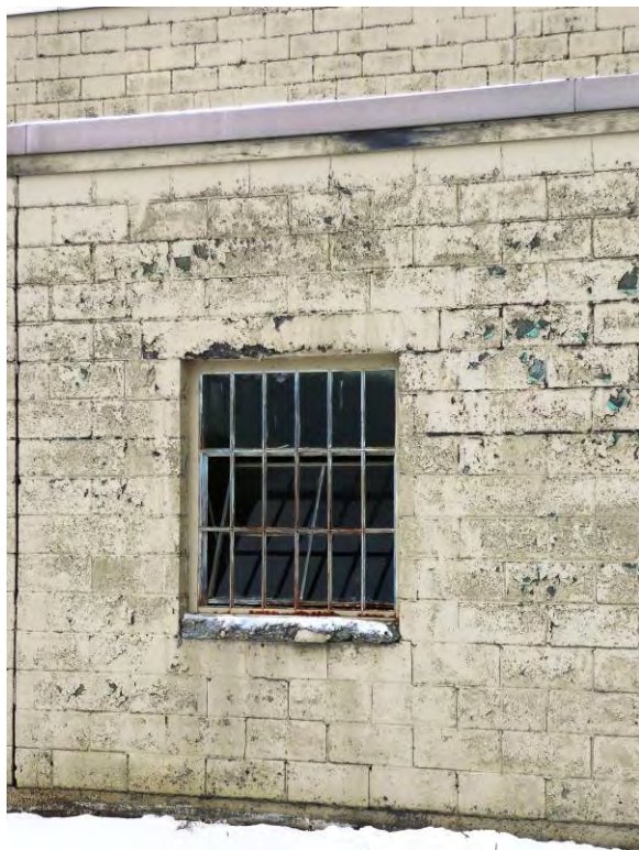
Building 1800 – original steel hopper window with a security grate on the west elevation
