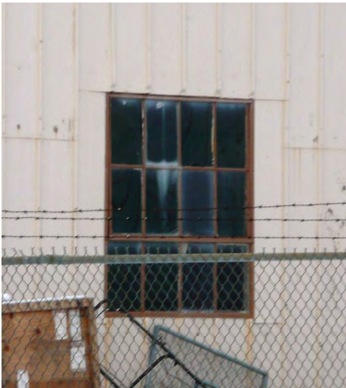
Building 1445 – close-up of original twelve-pane steel awning window on the south elevation
