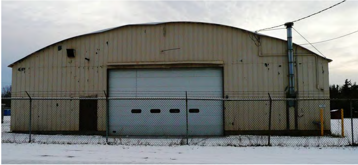
Building 1445 – east elevation
