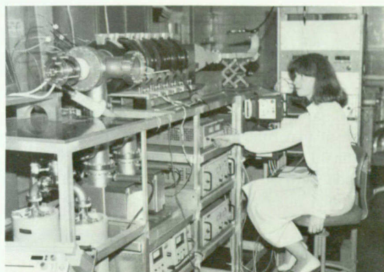
CUSPTRON: A compact high-power microwave tube, developed at NSWC.
