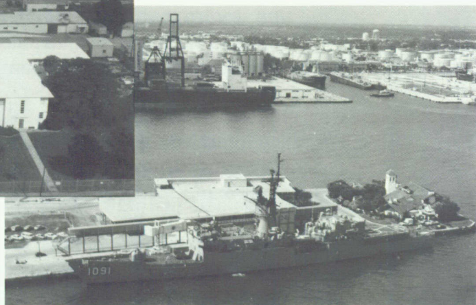
The Port Everglades harbor, across the ship channel from NSWC's south jetty, accommodates large ocean-going military and commercial vessels.
