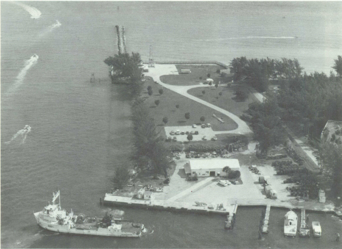
Leaving its pier at the south jetty, work boat RSB-1 enters the Port Everglades ship channel.
