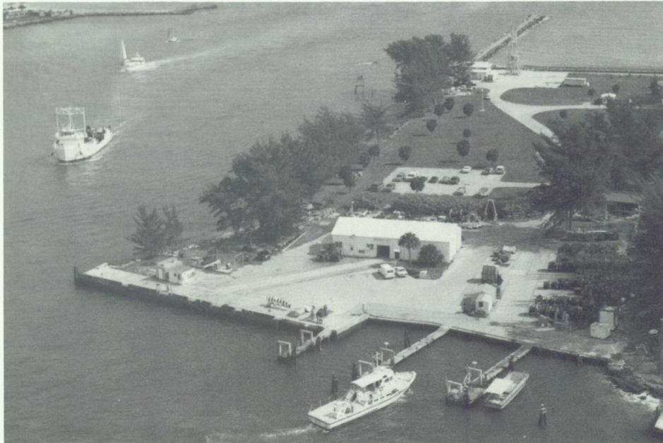
Aerial view of NSWC's marine facilities.
