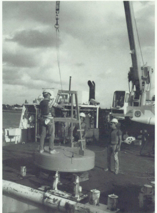
Crew readies buoy on deck of work boat RSB-1.
