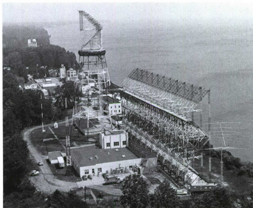
Figure 4. NRL's MADRE HF radar, on the western shore of the Chesapeake Bay, is continuously steerable from 47^\circ to 107^\circ true bearing, with a beamwidth of about 13^\circ at 13.5 MHz. The two rows of horizontally polarized dipoles, one above the other, can be fed in phase or anti-phase for moderate elevation angle control. It was used as the transmitter for the surface-current measurement program.
