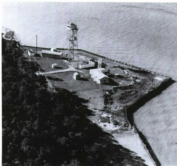
NRL's Tilghman Island test site
