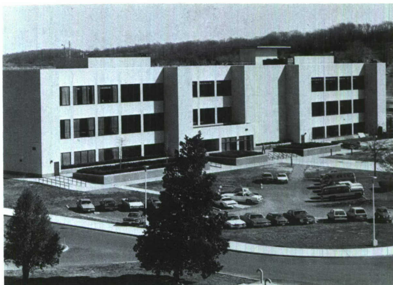
The new laboratory for electronic warfare research in the final stage of construction
