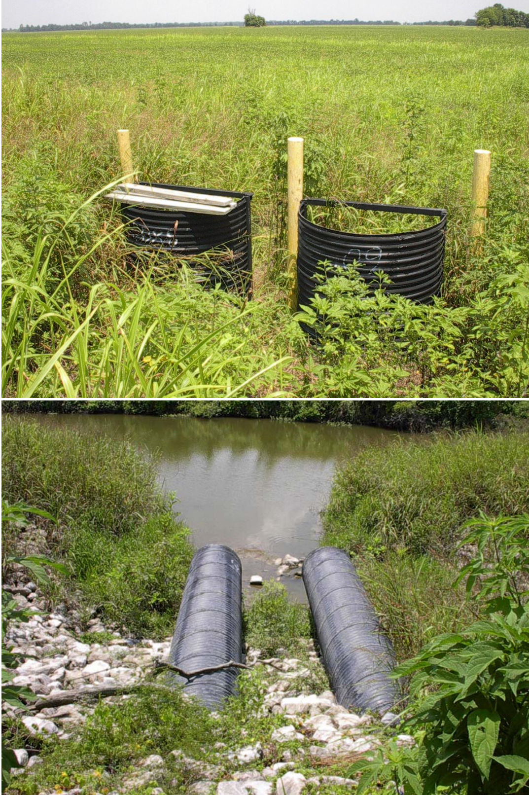
Figure 8. Drop pipes constructed in agricultural fields reduce erosion and sedimentation in streams.
