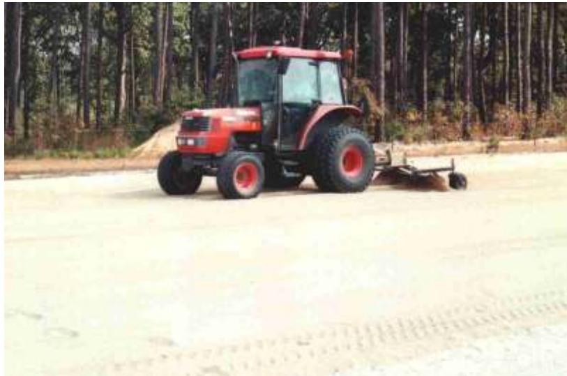
Figure 19: Raking of Sand at Test Site 3
