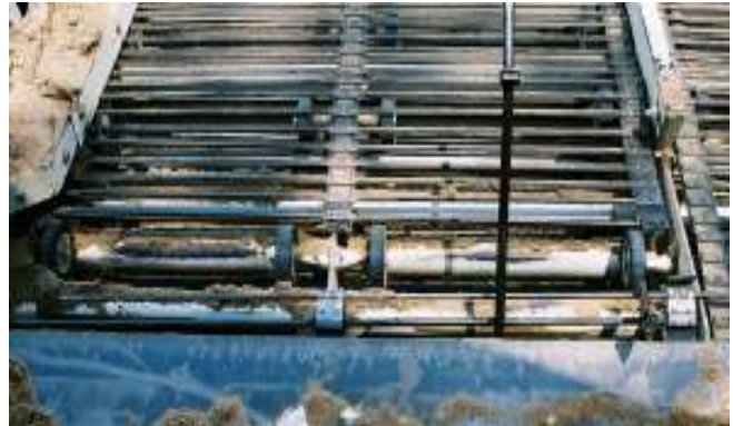
Figure A-23: Broken Sifting Belt
